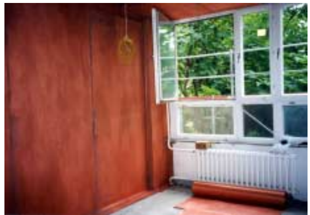
Installation of a shielding wall paper
