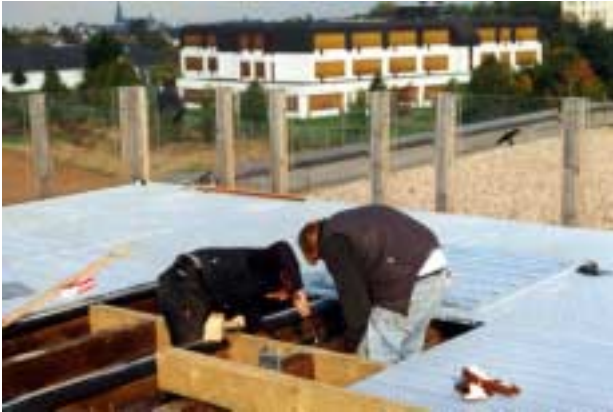
Installation of an Open Test Site
